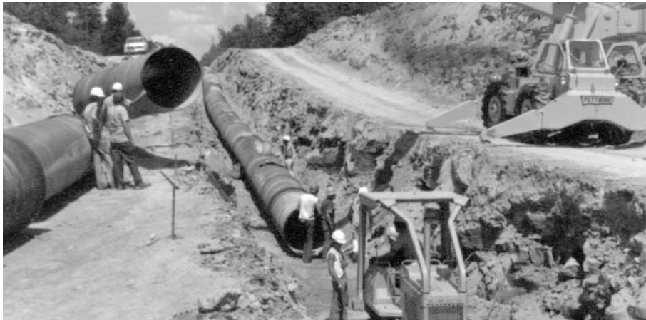
The liberal allowable deflection in the Fastite Joint facilitates pipeline installation with sweeping horizontal or vertical curves without the use of fittings.
