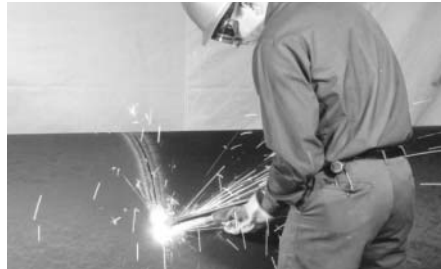
Cutting ductile iron pipe with torch.
