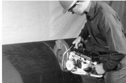
Cutting ductile iron pipe with abrasive wheel.
