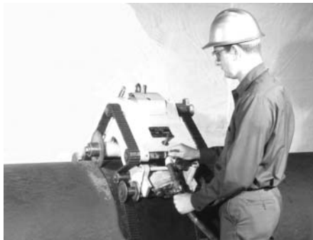
Cutting ductile iron pipe with milling cutter.
